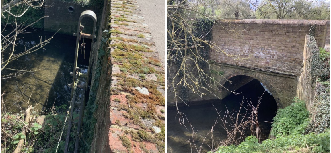
Figure 28: Weir (left) and Bridge (right), High Street
