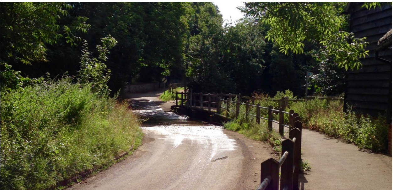
View 2: East along Church End over the ford
